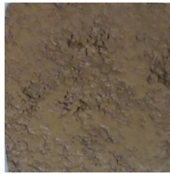
(a) rill erosion
